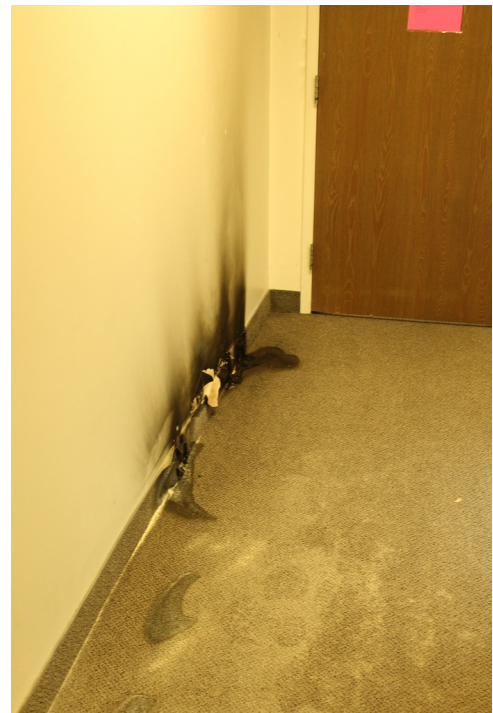
Looking at the head of the fire damage from inside the hallway. A garbage bag likely swung around the automatic door as it opened, was ruptured between the door and the wall, and started leaking an alcohol-like liquid.
